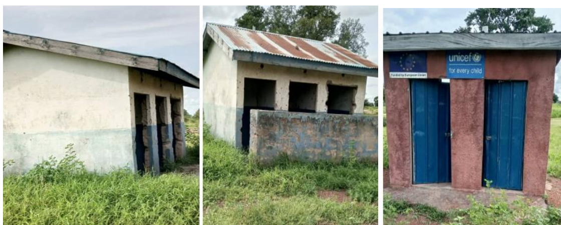
Figure 14: Photo of a public sanitation facility in Aweil East County
